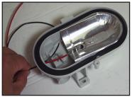
2 Punch out the required number of wire holes required for installation. Three holes are provided. Holes are scaled for 1/2" conduit. Insert positive and negative wires.
