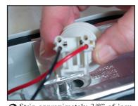
Strip approximately 3/8" of insulation off of wires and insert wire ends into the bulb recepticle. Wires will be locked in once completely engaged. Note that four wiring connectors are supplied on the bulb recepticle for multiple light circuits.
