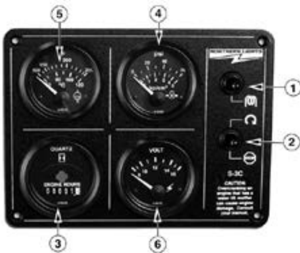
Figure 3-B: Series 3 Generator Control Panel
